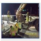
December 3 - Crews worked overnight to fill the bridge ends in prepara for base asphalt. This work eliminated the steel plates that had been covering the bridge/road joint areas for several months.
