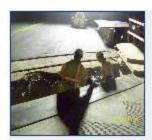
December 3 - As the fill is placed throughout the night, workers use a "jumping jack" to compact the material. When the backfilling and comp operations are done, base asphalt is placed. Final paving of these are take place later, in conjunction with final paving of the West Nursery R bridge approaches.
