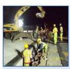
December 3 - While the area is backfilled, another crew works to cut a remove the tops of the steel "sheet piles" that were driven deep into th ground to stabilize the road bed and create a safe work area.
