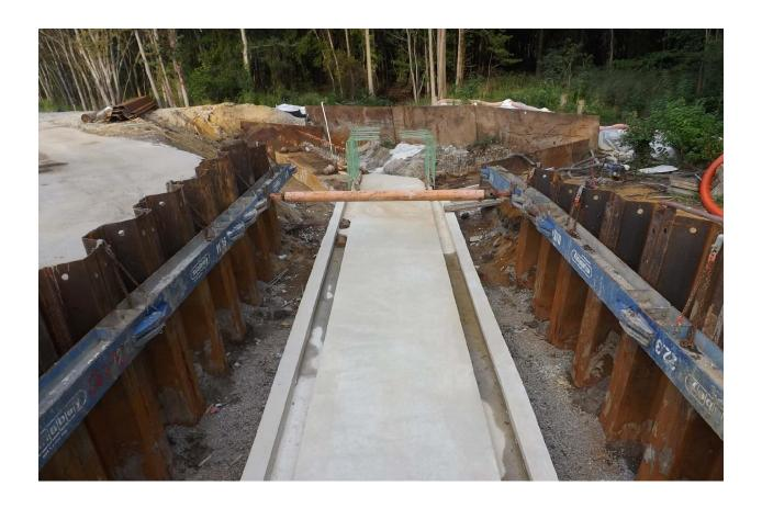
The floor of a large box culvert system takes shape along the northbound lanes of US 301. This structure will eventually carry a stream from the wooded area under US 301. A series of similar culverts is being constructed along southbound US 301 to provide stream continuity through the new interchange and roundabout areas.
